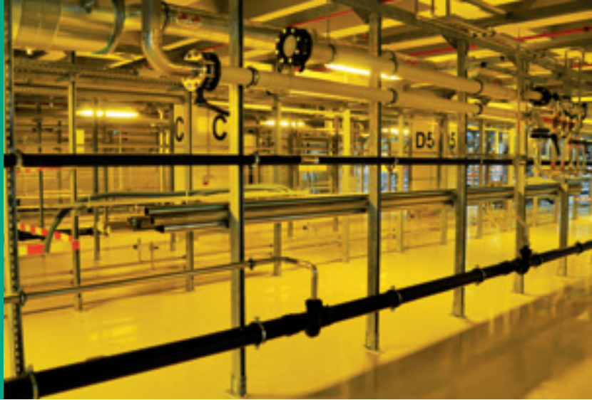
Clean sub-fab in the new cleanroom building
