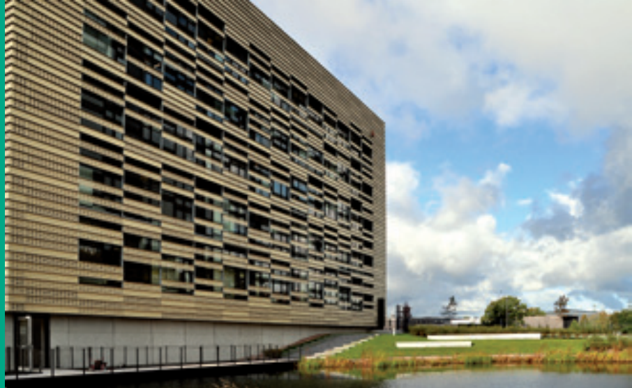
The new ISIT cleanroom building
